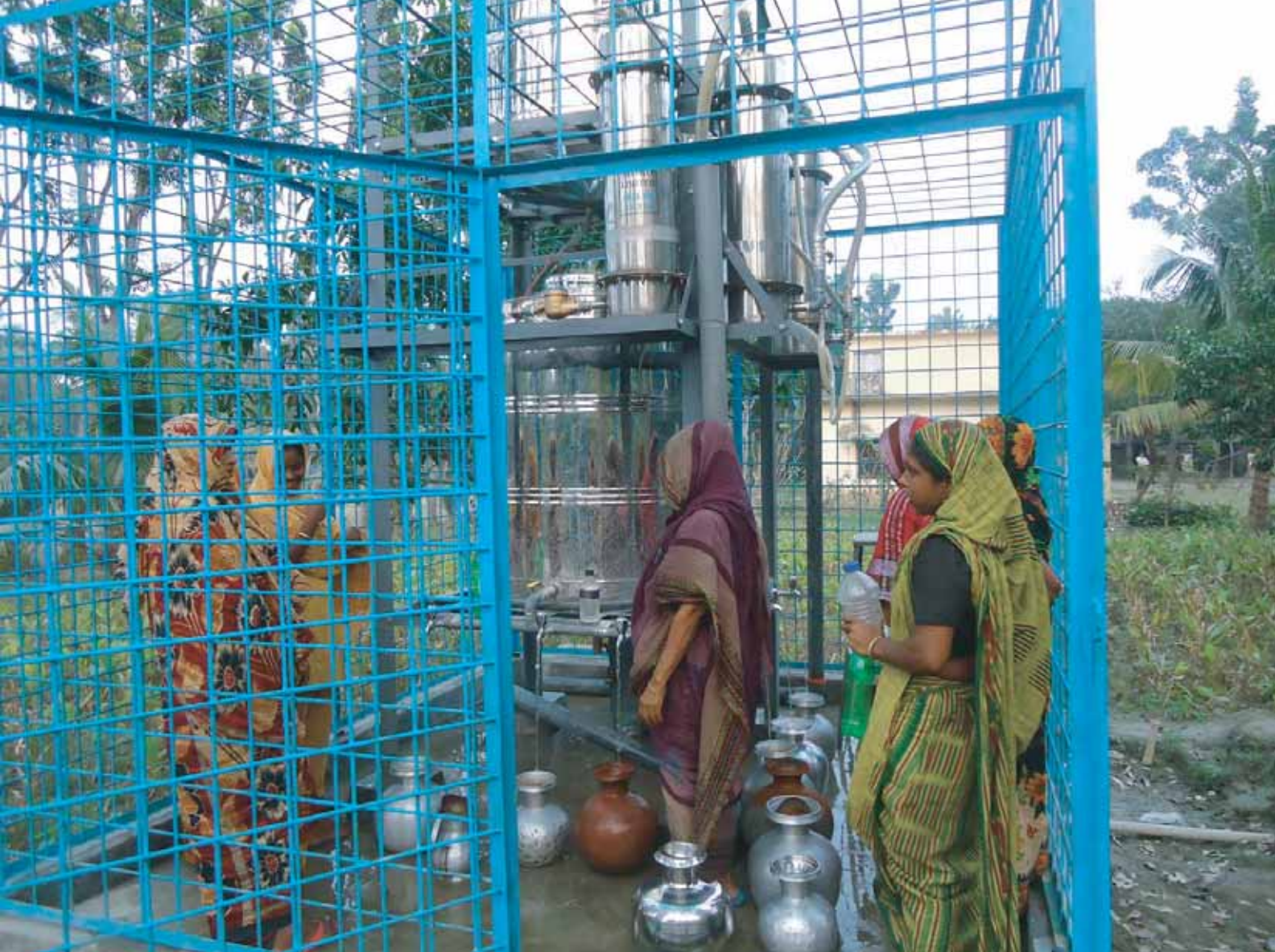
Arsenic Removal 'Sidco' plant at Chougacha in Jessore
